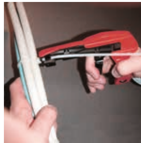
Tighten the tie till the complete fixing of the cables.
