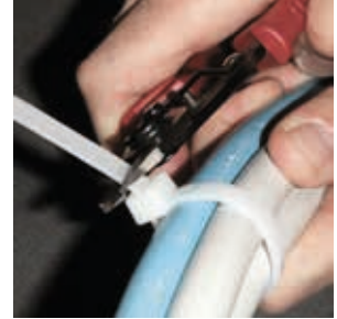
Cut the exceeding part of the tie with the tool, leaving a few mm length as safety.
