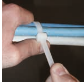
Tighten manually the tie till the complete fixing of the cables.
