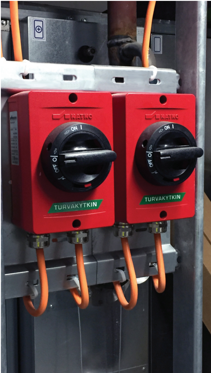
KATKO Firerated switches at Keilaniemi metro station in Espoo, Finland
