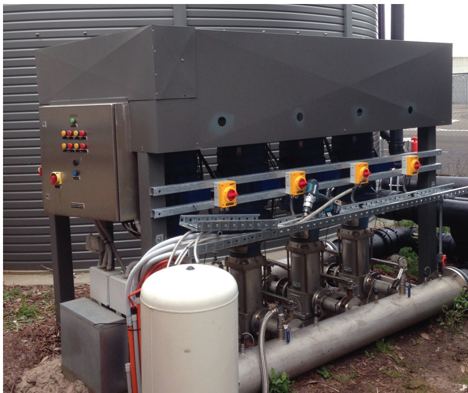
KATKO EMC safety switches installed to a water purification system at the Sydney International Airport.
