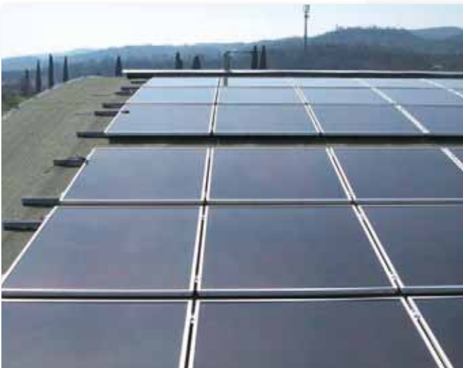
Industrial sheath arched roof. Direct application of the hot galvanized PRF with Butyl gasket.
