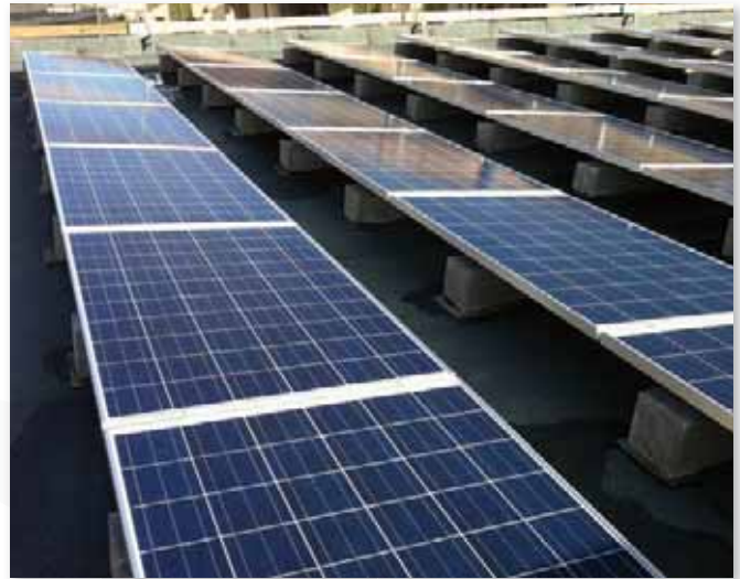
Horizontal panel with Flat ballast.
