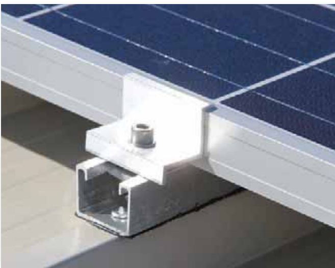
Metal decking roof with FVT5120.
