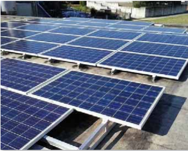
Triangle triple horizontal ballasted.
