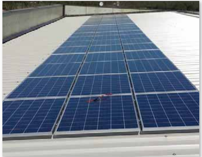
Metal decking roof with FVT5000.
