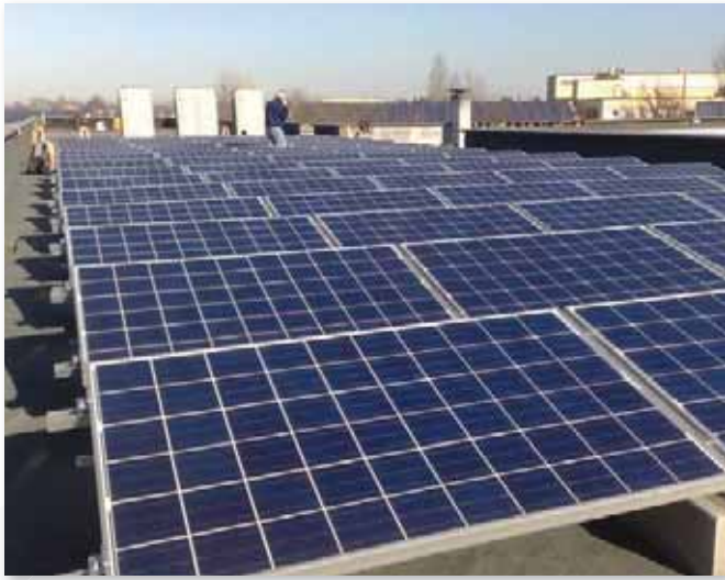
Roof with ballast application.
