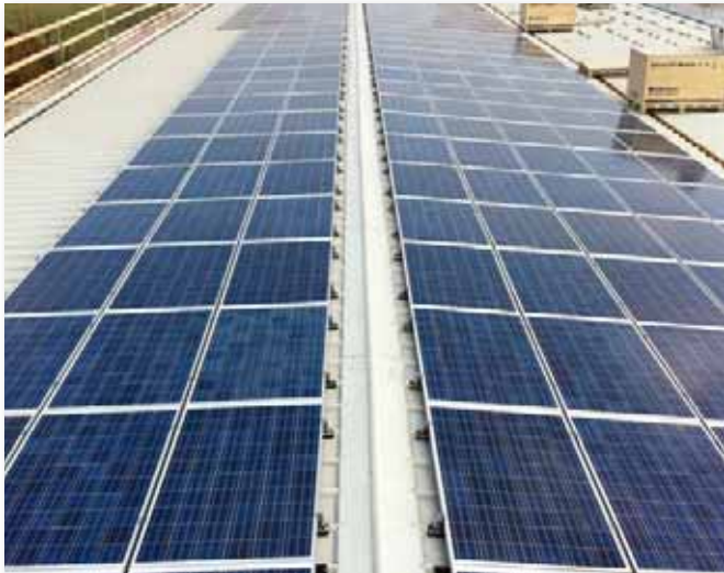
Metal decking roof with FVT5000.
