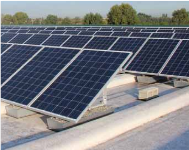
Triangle single vertical at 30° with ballast tanks.
