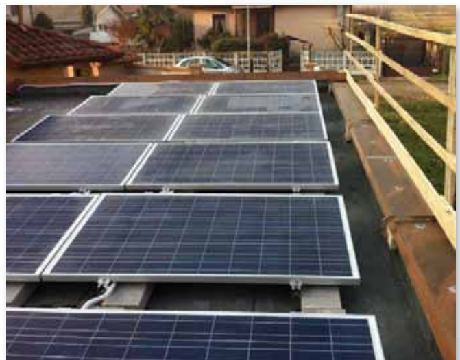
Flat ballast with horizontal panels.
