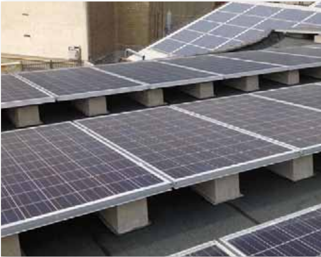
Flat ballast with vertical panels.
