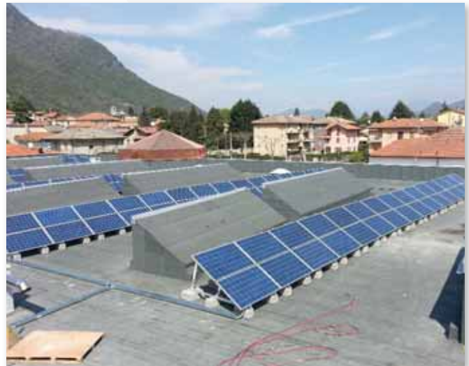
Triangle Double horizontal at 30° and ballast.
