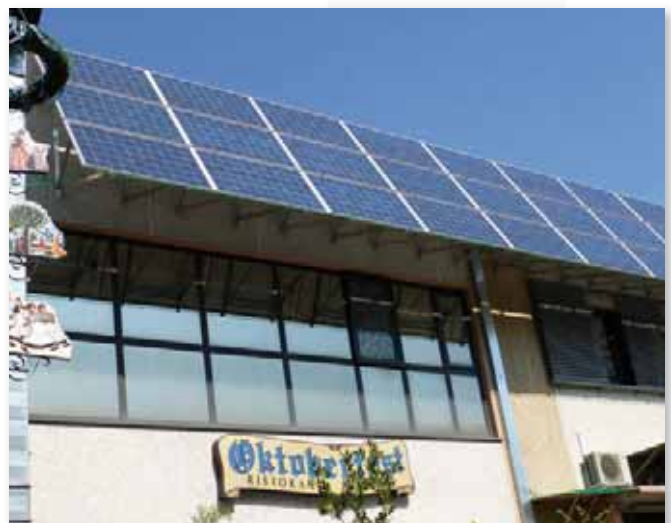
Sloping roofing structure.
