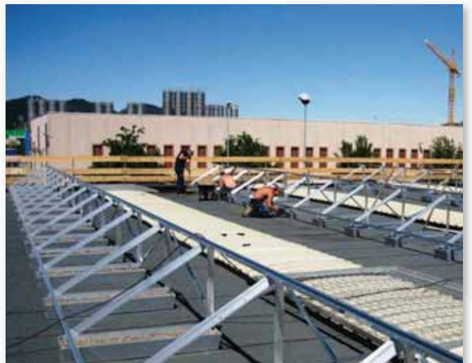
Flat industrial roof with sheath. Application with ballast tanks FVT1455 and triangles at 30° FVT1511.
