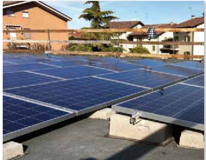
Flat ballast application.
