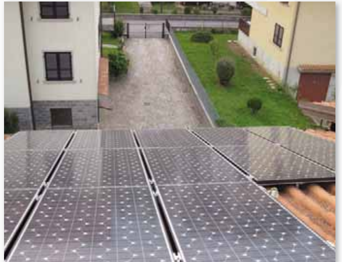
Sloping roof with tiles. Application with stainless steel adjustable bracket FVT1256.
