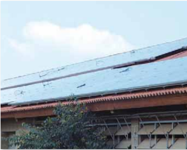
Sloping roof- asbestos recovery. Application with mill screws for wood FVT1315.
