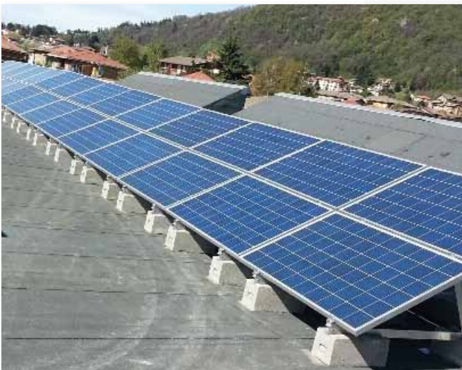
Triangle double horizontal at 30° ballasted.
