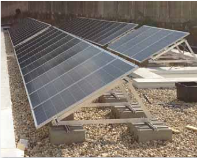
Triangle single vertical at 30° ballasted.
