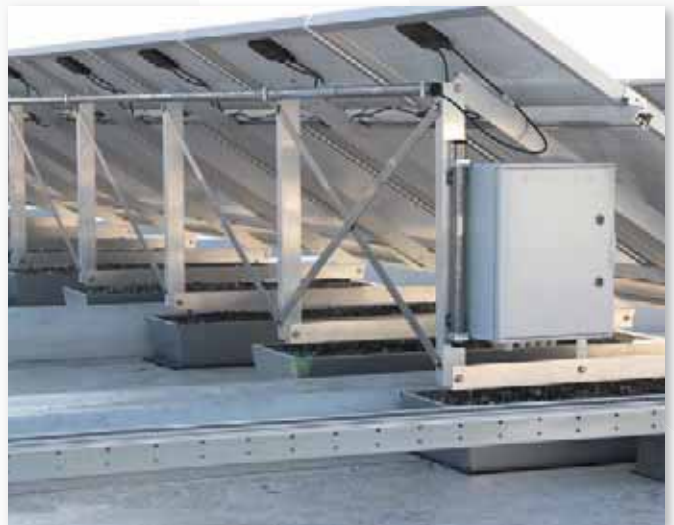
Triangle single vertical at 30° with ballast tanks.
